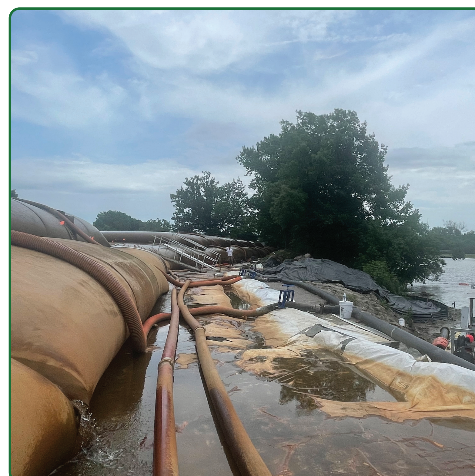
Sediment dewatering operations in progress.
